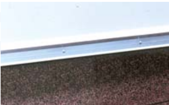
T-Bar aluminium termination bar
